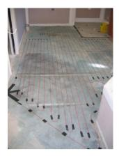
The hot/cold joins between the heating cable (blue) and the cold cables (black) must be embedded within the floor. Run the cable around to the opposite side of the heated space, then zig zag the cable back towards the termination point sticking down at the ends only until you are satisfied that reasonably even spacing is achieved.
